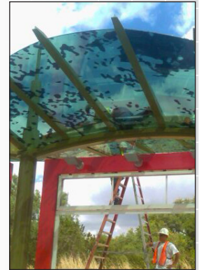
Fresco decorated glass canopies are installed at four train stations in Austin, TX.
